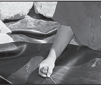
Fig. 11 Mark the outer perimeter of the skimmer opening on the liner; then mark a second box 1.5" inside of it. Cut out at inside mark.
