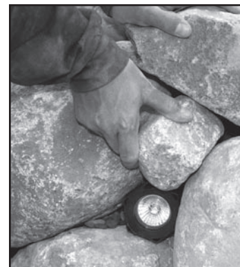
Fig. 18 Set your underwater lights in between your boulders so they are hidden from view.
