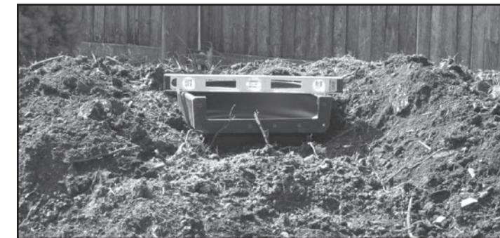
Fig. 6 Soil backfilled around the filter creates a planting berm.
