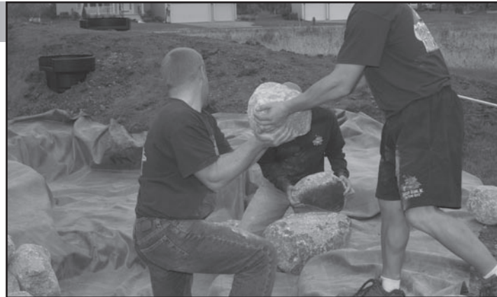
Fig. 16 Starting at the bottom, set the largest character boulders first then fill in with the smaller ones.
