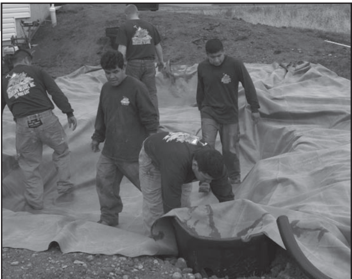
Fig. 9 Place the liner on top of the underlayment following the same installation procedures. Make sure liner is positioned in such a way that allows it to extend and completely cover the opening on the BIOFALLS® filter.
