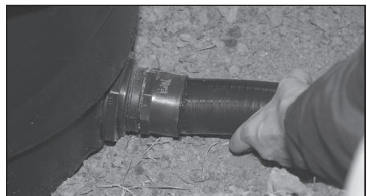
Fig. 4 Finished bulkhead assembly.
