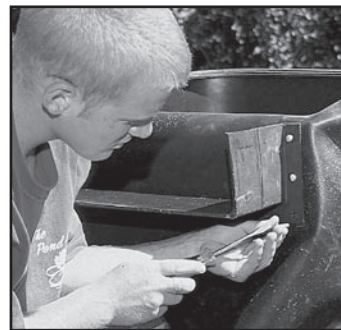
Fig. 7 Tighten the screws just enough to thread into the inserts.
