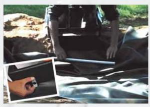
Run the protective underlayment in the pond and up the stream (if one is installed). The underlayment should overhang the stream bed and be up to the bottom of the filter box. Lay the liner in the pond over the underlayment. Work as many wrinkles out of the liner as pos-
