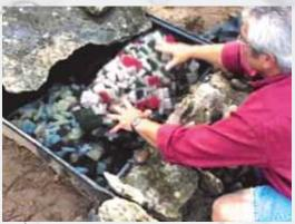
Stack stones up the front of the falls filter to conceal the filter box and liner. Additional stone can be added on top, just below the lip, to
