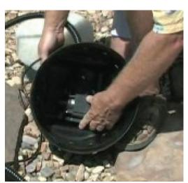
Place pump in bottom chamber of filter. We recommend EasyPro mag drive pumps up to 850 GPH.
