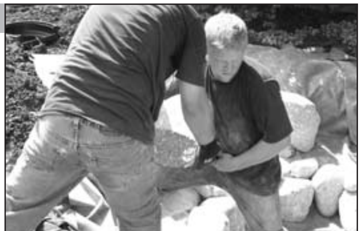
Fig. 21 Starting at the bottom, set the largest character boulders first, then fill in with the smaller ones.
