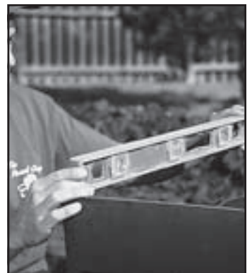
Fig. 6 Level the UltraFalls™ filter side to side as well as front to back.
