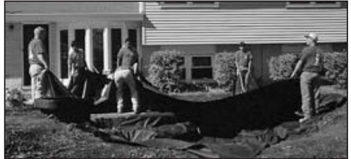
Fig. 13 Lay the underlayment and the liner into the excavated pond and conform to the contours and the pockets.
