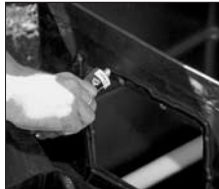
Fig. 19 After alignment, remove faceplate and apply silicone sealant.
