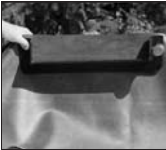
Fig. 27 Make sure you have a few inches of slack liner along the front base of your biofilter box
