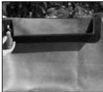
Fig. 32 Reattach the waterfall lip and liner.
