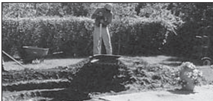
Fig. 10 Soil backfilled around the UltraFalls™ helps hide the filter and creates a planting berm.
