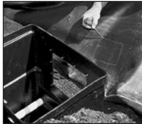
Fig. 16 Mark the skimmer opening on the liner and cut an area 1.5" inside that mark.
