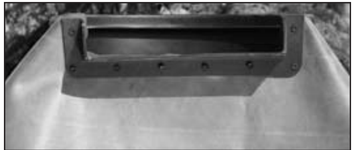
Fig. 33 Install the rest of the screws and remove extra liner, using the waterfall lip as a guide.
