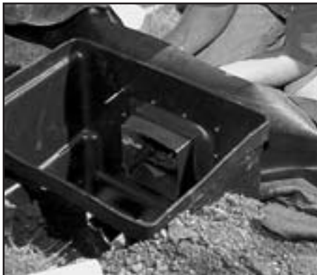
Fig. 18 Using an awl, poke holes through the liner at screw holes; temporarily screw top corners into place.
