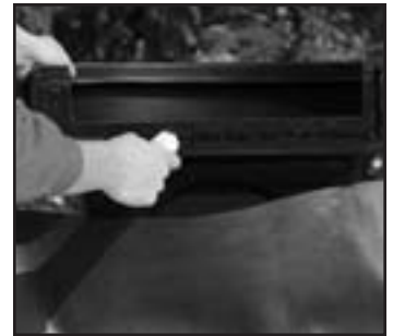
Fig. 30 Place a thick bead of silicone across the insert nuts.
