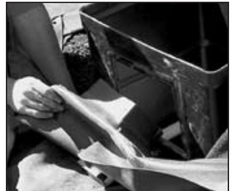
Fig. 20 Carefully replace the skimmer faceplate into the silicone-lined opening.
