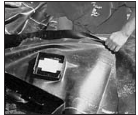
Fig. 17 Place skimmer faceplate through liner and place into skimmer for alignment.
