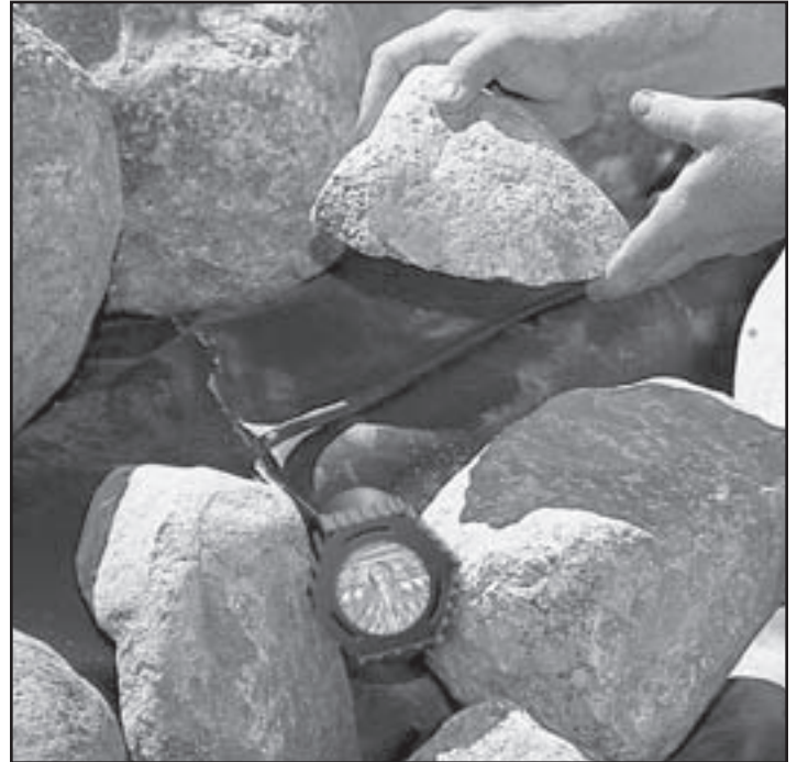
Fig. 23 Set underwater lights between boulders so they are hidden from view.
