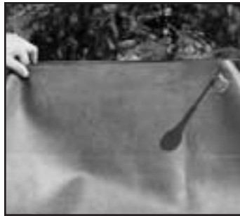
Fig. 28 Poke holes in the liner all the way through to the inside of the filter box.
