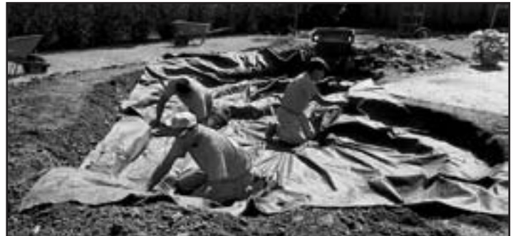
Fig. 14 Place the liner on top of the underlayment, following the same installation procedures. Make sure liner is positioned in such a way that allows it to extend, and completely cover, the opening on the UltraFalls™.
