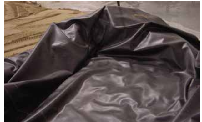
Sculpt and compact dirt in stream area before installing liner
