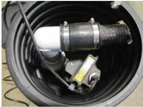
Do not overtighten discharge assembly while installing pump into vault.
